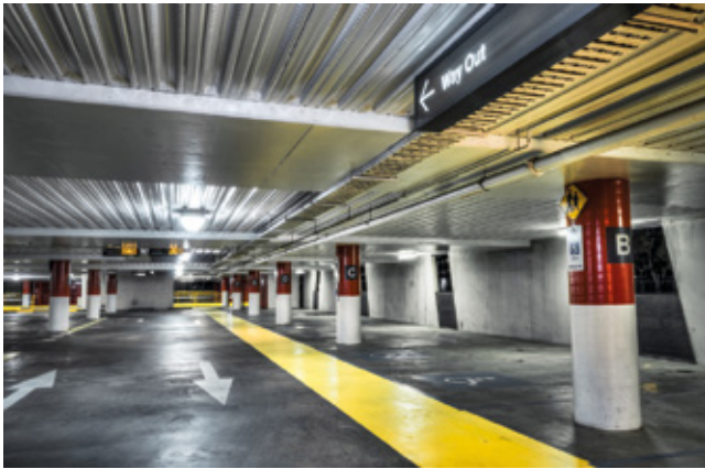
Enclosed car park
